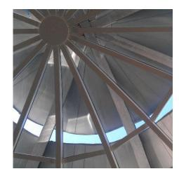
with a tough end outer pane, argon filled cavity and toughened/laminated low e inner which not only gives great thermally and light transmittance properties but also complies with a burglar resistance rating P4A to EN356. Whilst an option for a dual curved dome can be supplied clients must be aware to the greatly increased lead time and cost over the more commonly specified single curved option.
